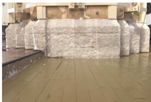
3.att. Kolonnas austrumu puse ar lignīna kompresēm/ The east side of column with lingnin compress
